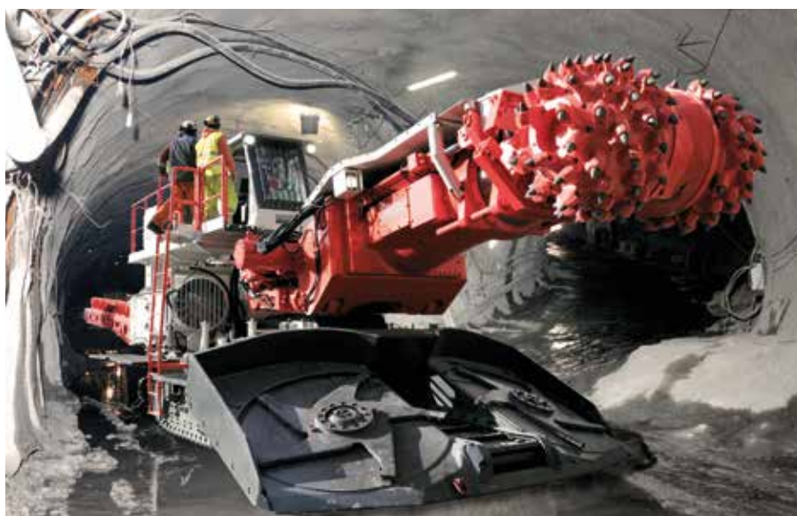
Tunnelling roadheader © Sandvik Mining and Construction GmbH
