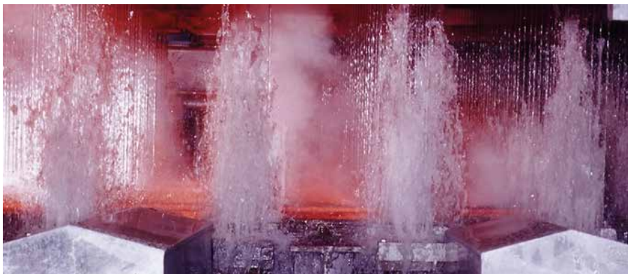
Accelerated cooling line in operation
